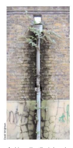
An obvious problem with a simple remedy: no special skills or equipment are needed to remove this blockage and allow the water to flow freely into the hopper again
