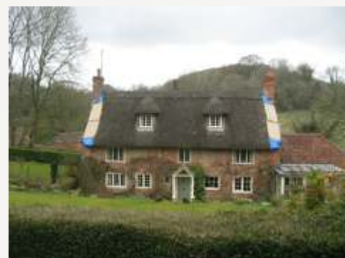
Park Cottage with temporary verge repairs
