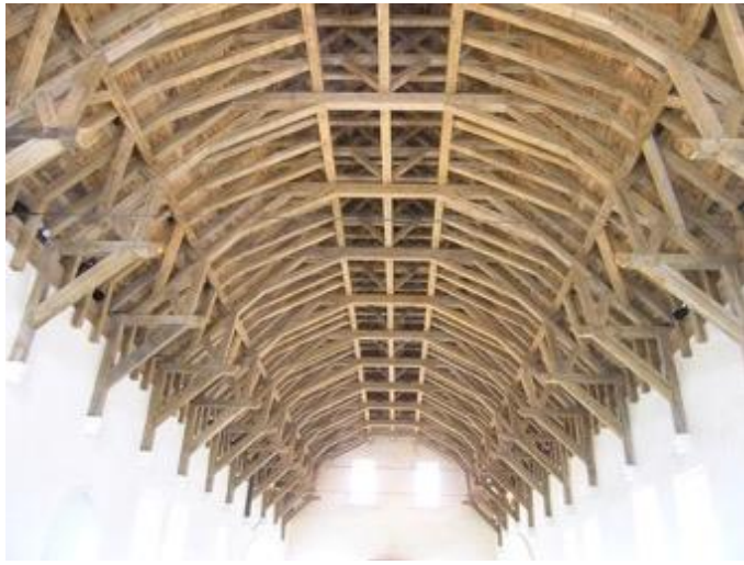
Stirling Castle Hammer beam roof
