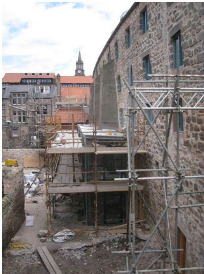
Photo of Dewar's Lane Granary restoration by Ken Hutchinson
