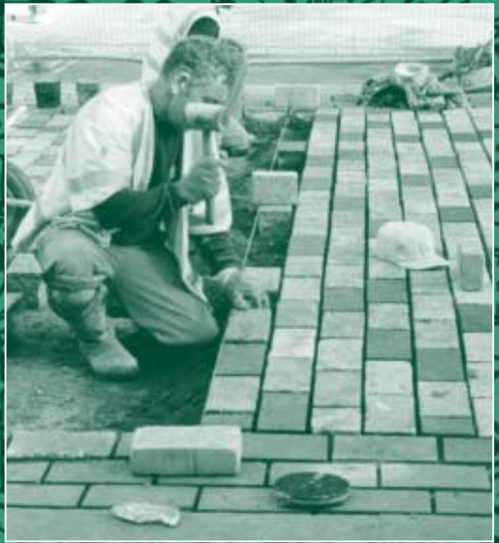
Top quality sett-laying in Halifax town centre. Contractor: Tarmac Ltd
