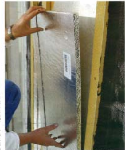
Installing the vacuum insulated panels in the Munich building.
