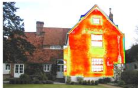
There is no evidence of any timber frame surviving within the west elevation. There is a very faint indication that the tie beam and collar of the roof truss have been retained within the masonry.
