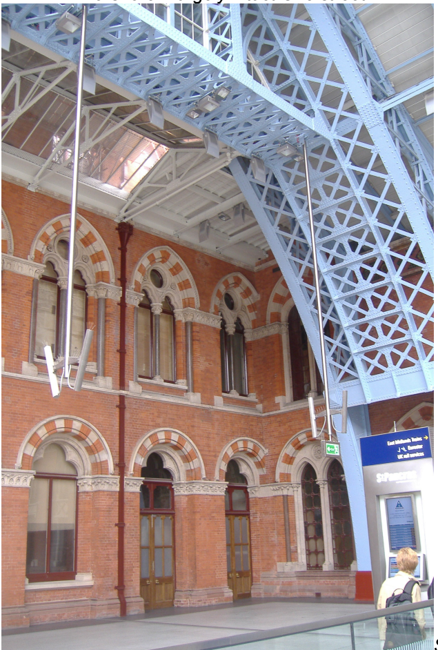
t Pancras. Contrast between Scott's Venetian Gothic and Barlow's more functional wrought iron
