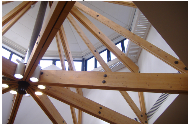
That roof construction!
