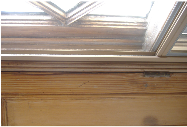
Mere Hall – interface between Storm Windows secondary glazing and early C19 'lattice' sash
