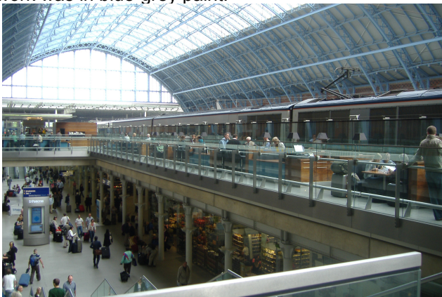
Trainshed, with light well cut into the former Goods Cellar
