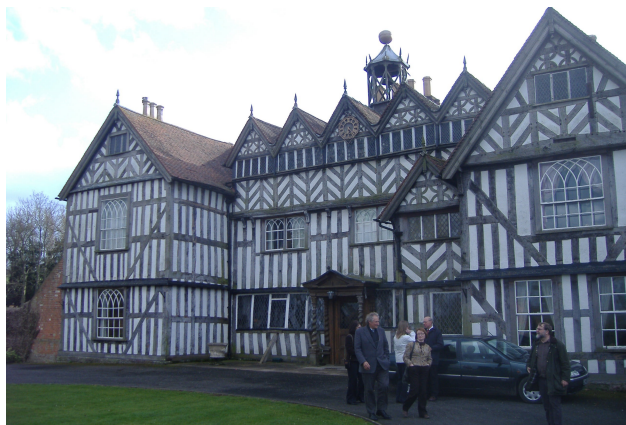
Mere Hall – main entrance front
