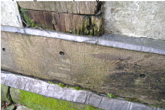
Flashband – and moss growth demonstrating water retention
