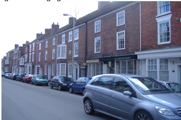
Eastern High Street, Pershore. Continuous Georgian brick!
