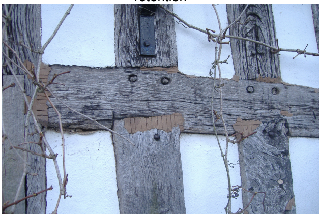
Mortar patching to framing
