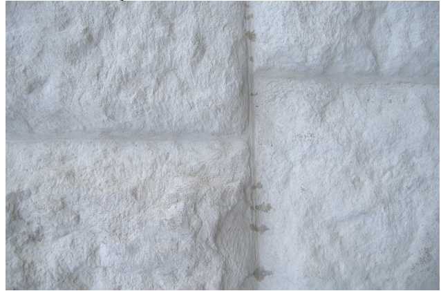
The new coating
