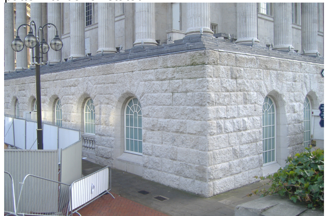
Plinth with lead-sheathed steps above
