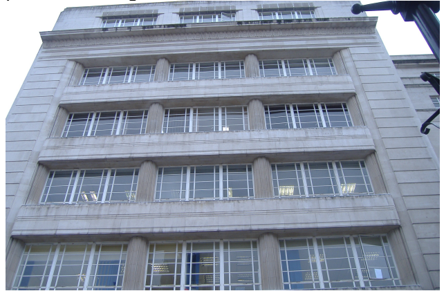
Neville House – with original steel windows
