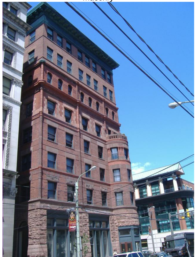
Brooks Building. Washington Avenue, Scranton. Chicago-style high-rise in the Richardson manner, clad in pinky-brown stone. Some carved decoration reminiscent of Louis Sullivan’s work.
