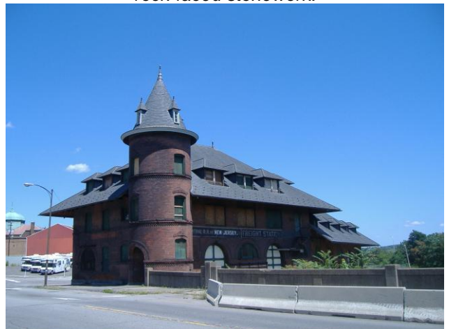
Railroad Goods Station, Lackawanna Avenue, Scranton. Arts and Crafts Gothic
