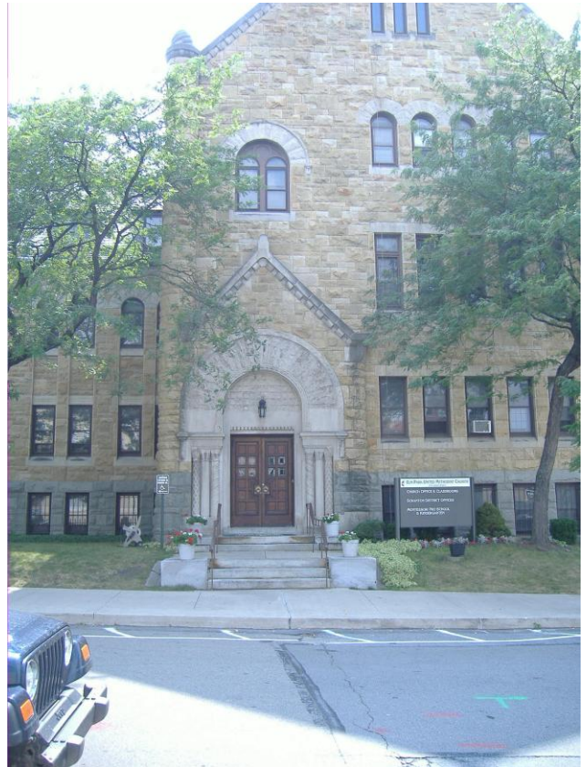
Detail of Elm Park Baptist Church, Scranton. An essay in Richardsonian Romanesque with rectilinear rock-faced stonework.
