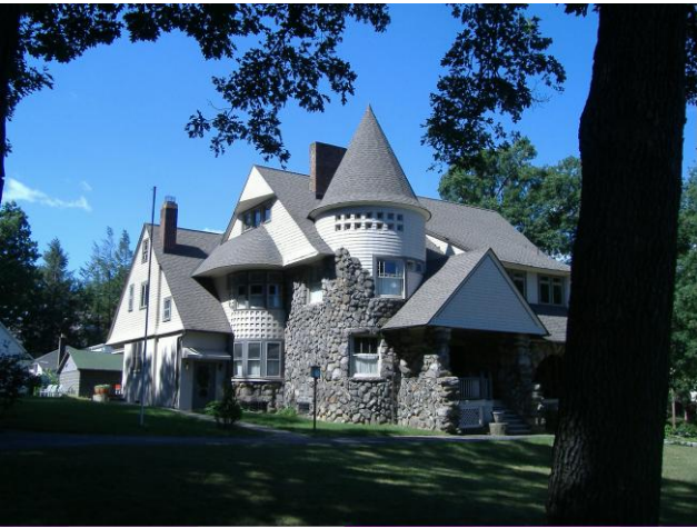
Mine Baron's Villa, Green Ridge, Scranton. Arts and Crafts design combining partial rubble facing with timber framing and cladding.
