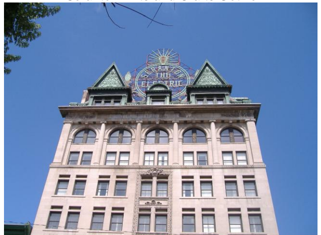
Art Deco "Electric City" building, Linden Avenue, Scranton. Terracotta clad.
