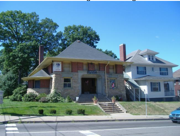
Green Ridge Public Library, Scranton Elegant Arts and Crafts building after Richardson, with stone-faced ground floor and brick-faced first floor. Deep eaves.
