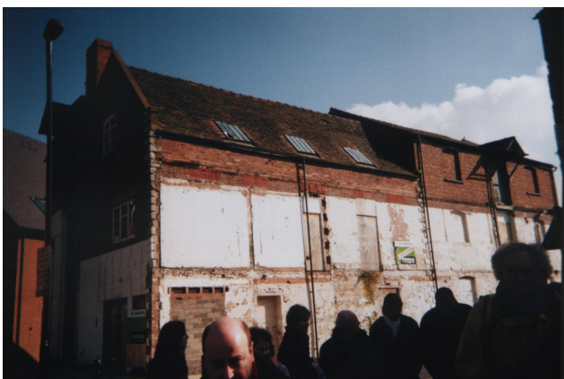
West face of early C18 town house converted to a warehouse. Guildhall immediately behind
