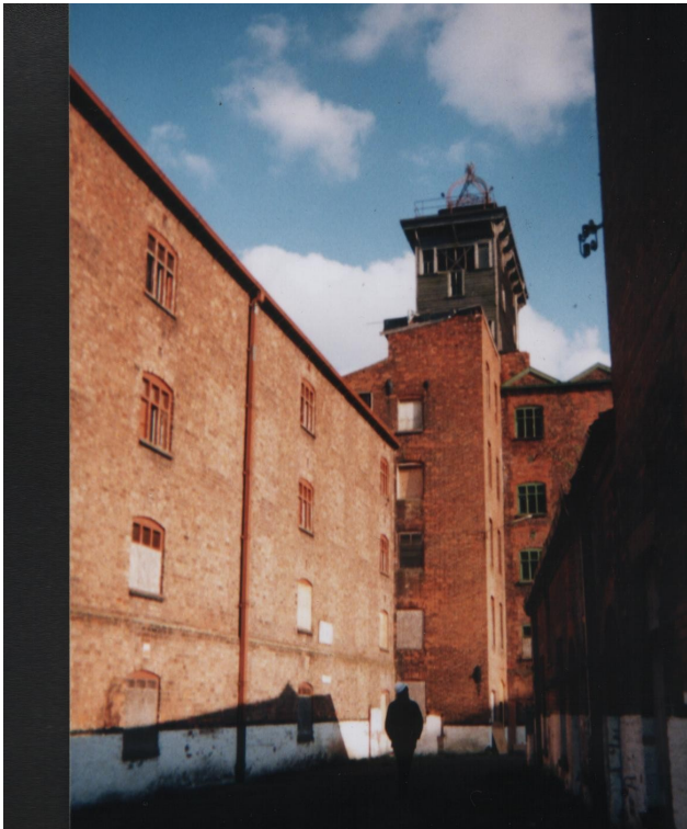
View from north, showing north wing and centre 'belvidere' turret. Grain store in shadow to the right.
