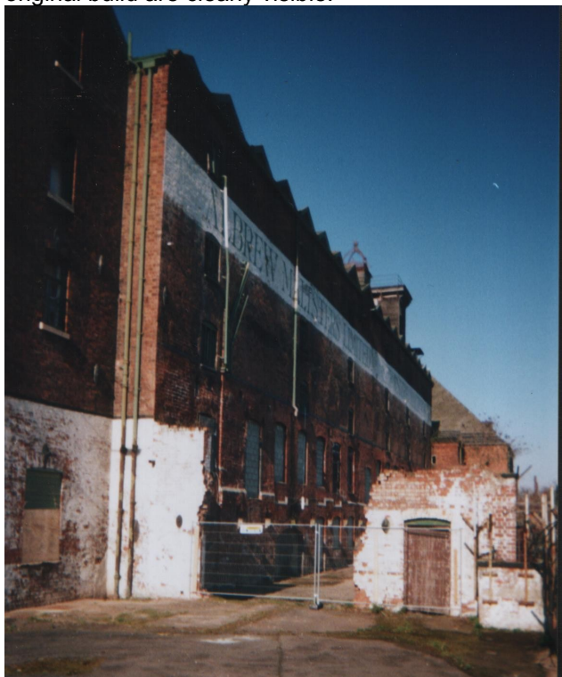
Tall main frontage, topped by a row of gables reflecting the unexpected roof form.
