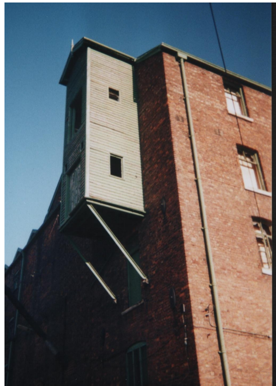
Diddington Flax Mill. NW corner of main block, showing close-boarded hoist.
