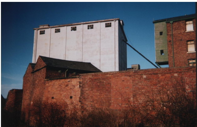
View from the west outside the curtilage. Boundary wall and ancillary stabling. C20 concrete silo to left and part of main block – with attached hoist – to extreme right.
