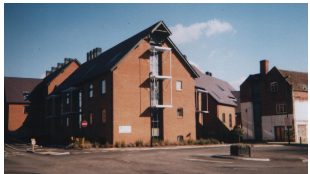
Shrewsbury Guildhall from the west, indicating the 'industrial vernacular' style used
