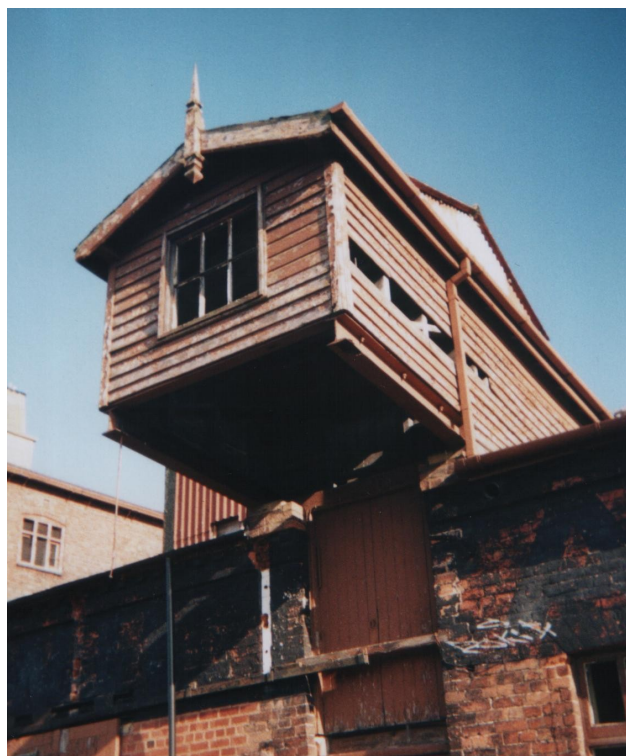
'Railway style' hoist to grain store. There are two of these.
