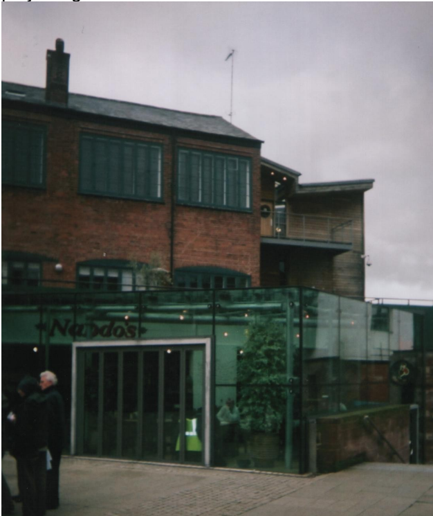
Ribbon factory. Original, centre left. Upper right, service turret. Below, 'glass box' restaurant.
